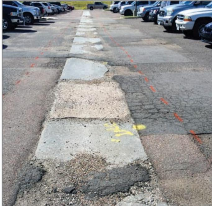
The removal and replacement of a concrete drain pan and an asphalt patch – shown here at a Century Link in Colorado Spring – are extremely common maintenance tasks in Colorado due to the climate.
